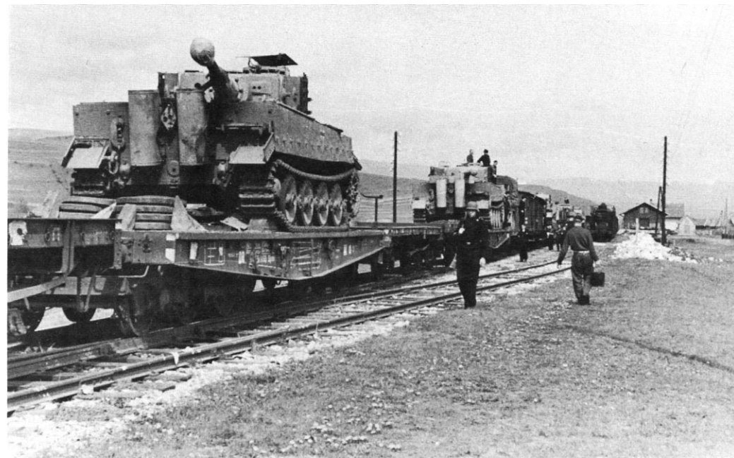
Tigers of Grossdeutschland arrive at a unit assembly point in Lithuania during August of 1944. These vehicles are overall Dark Yellow with a light pattern of Olive Green. The narrow transport tracks were placed back on the flatcars once the wide battle tracks were installed on the tanks. The side skirts are stored under the tanks and the outside roadwheels are in front of the tanks on the flatcars.
