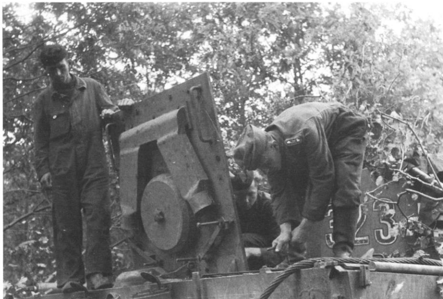
The crew of this Tiger has raised the rear engine cover to gain access to the engine compartment. Normally, repairs were made in rear areas and under cover to protect the immobile Tiger from detection and destruction by enemy aircraft.
