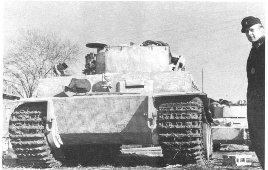
This mid-production Tiger is fully coated with zimmerit anti-mine cement. The open driver's and radio operator's hatches reveal the periscopes fitted to the hatch. This Tiger has also had the first outer road wheel removed to prevent jamming or obstruction of the track and sprocket.
