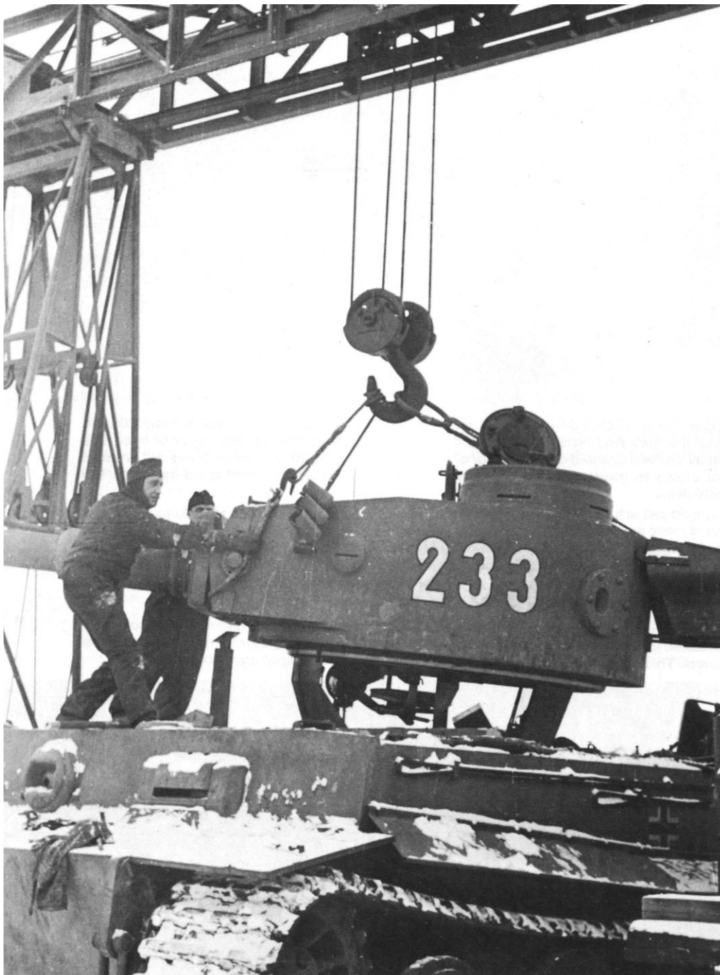
sPzAbt 503 received its first Tigers during late 1942 which were delivered in overall Dark Gray. This Tiger of the 2nd company is being overhauled in the Rostov area during early 1943 and has a PzKpfw III stowage bin fitted to the turret rear. Most Tiger units on the Russian front were forced to maintain their vehicles under very poor conditions.
