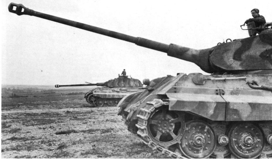
The early Porsche turret's front curved plate formed a shot trap that was a serious disadvantage for these vehicles. These early Tiger IIs have a complete coating of zimmerit anti-mine cement. The side skirts on the Tiger II were not thin sheet metal, but rather 5mm thick sheet that served as anti-bazooka skirts similar to those on late PzKpfw IVs.
